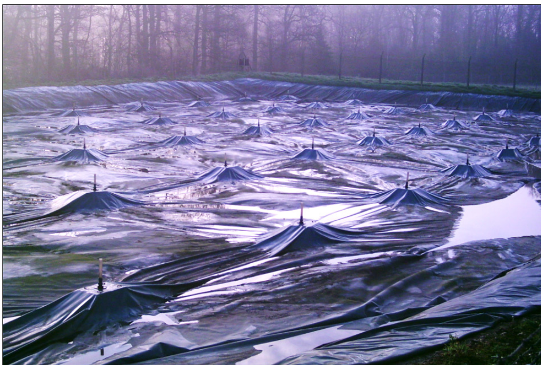
Figure 5: A floating plastic cover on an earth-banked slurry lagoon. Image credit: Defra
