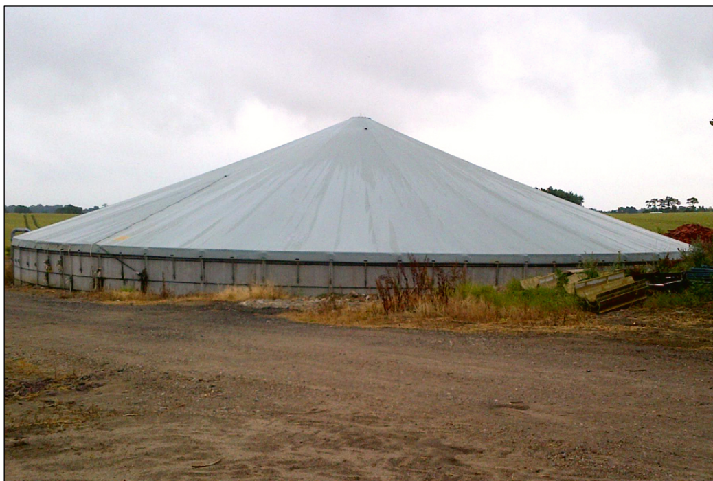
Figure 4: A fixed cover on a slurry tank.
