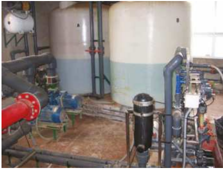
Head unit with typical A + B tank, large scale
