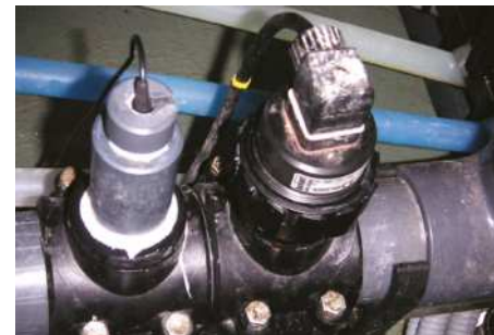
pH and EC meters at the head unit
