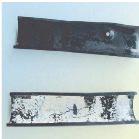
Scales in pipe before and after usage of Antiblock O™
