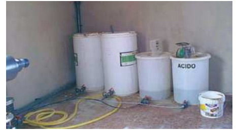
Head operating typical A + B tanks + specifics tanks for micronutrient and acid solutions, small scale
