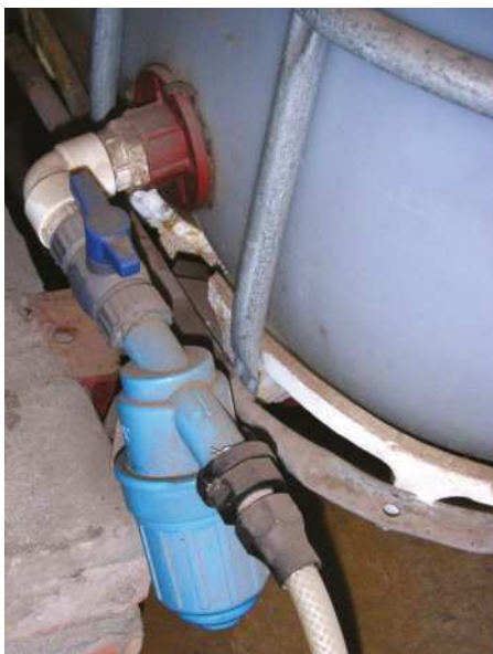
Screen filter used as control filter
