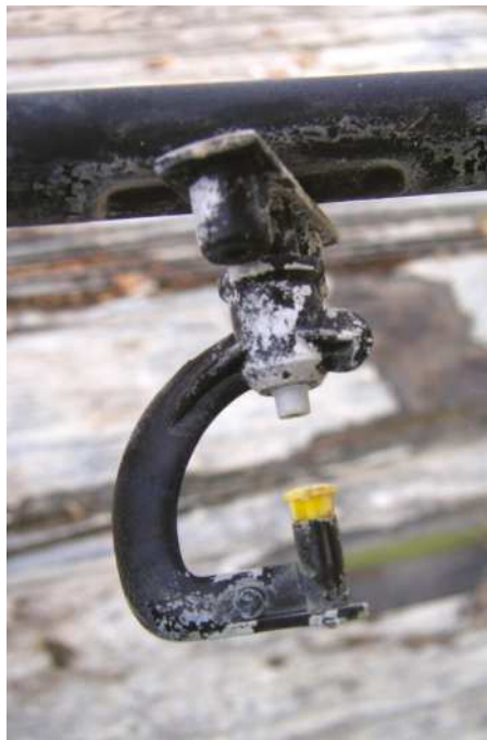
Scaling on a micro sprinkler
