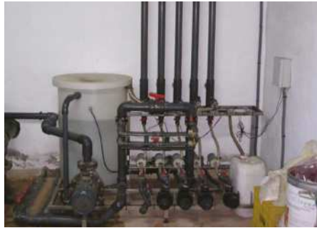
Head operating typical A + B tanks + specifics tanks for micronutrient and acid solutions, small scale
