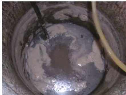
Tanks need to be cleaned before use as dirty tanks will result in problems
